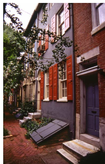
Trinity-style Row Home on Camac St.
